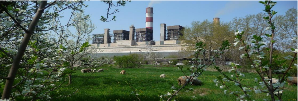
Figure 9. Branch Thermal Power Plants “Nikola Tesla”
