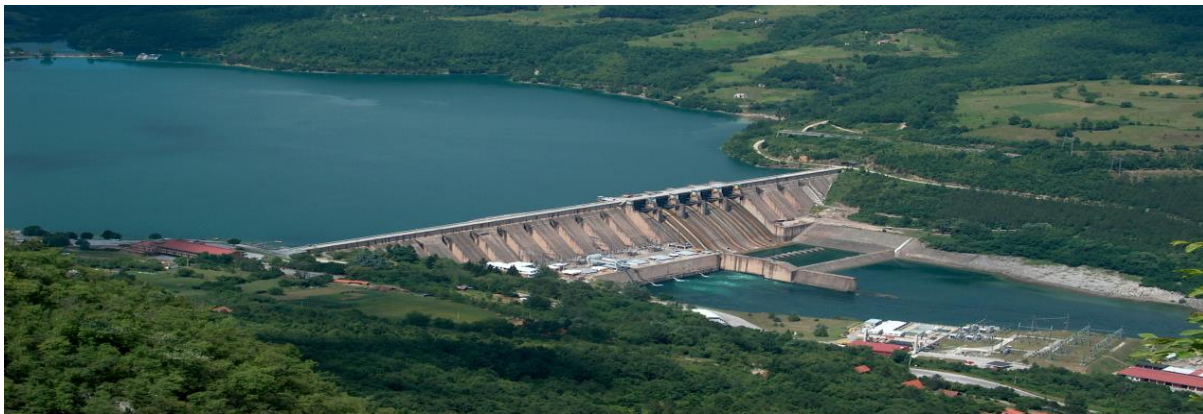
Figure 7. Drinsko – Limske Hydro Power Plant – Bajina Bašta
