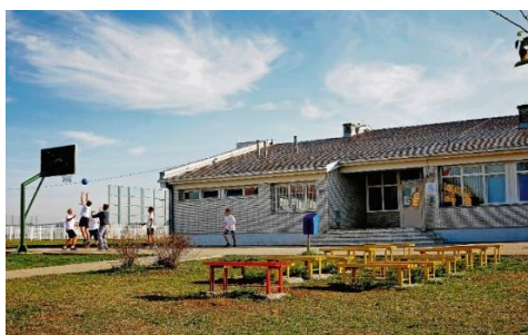
Figure 5. Works on the upgrade and reconstruction of the primary school in the settlement Crna Međa
